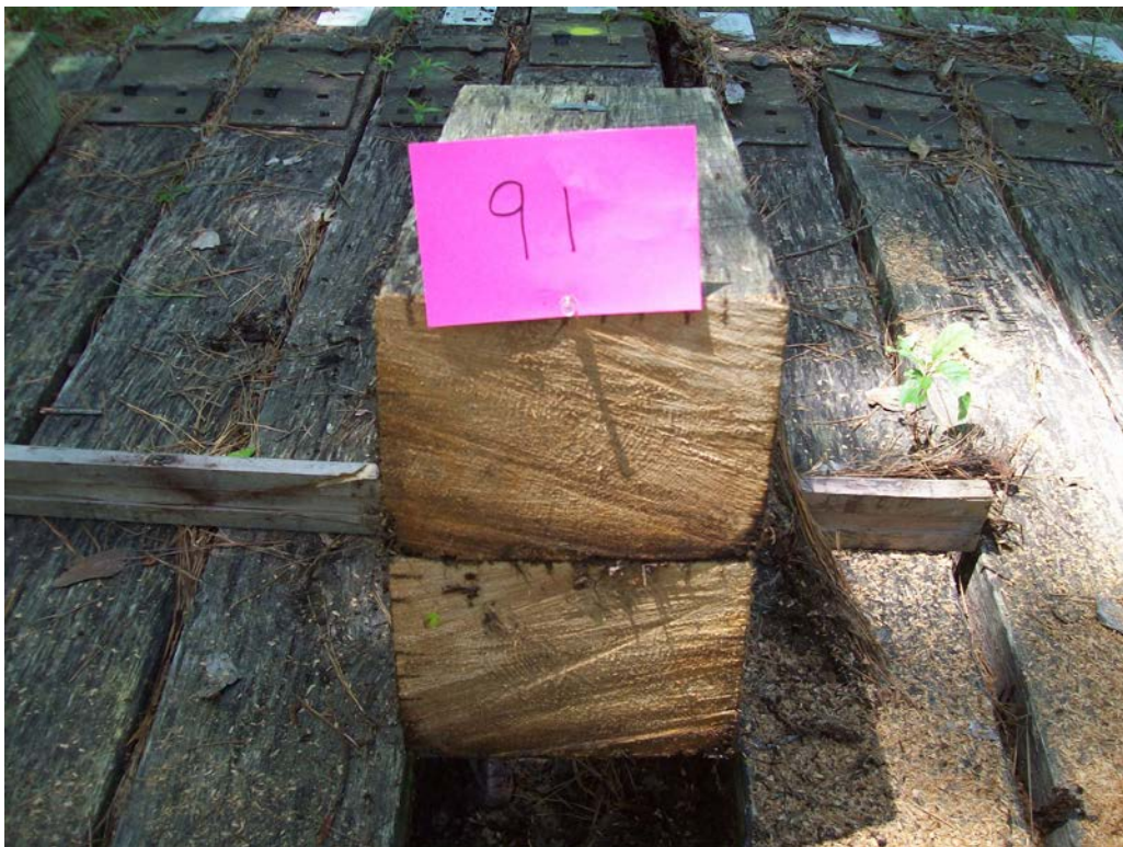
Figure 18 - Tie #91 (Lonza/white oak) decay on bottom.
