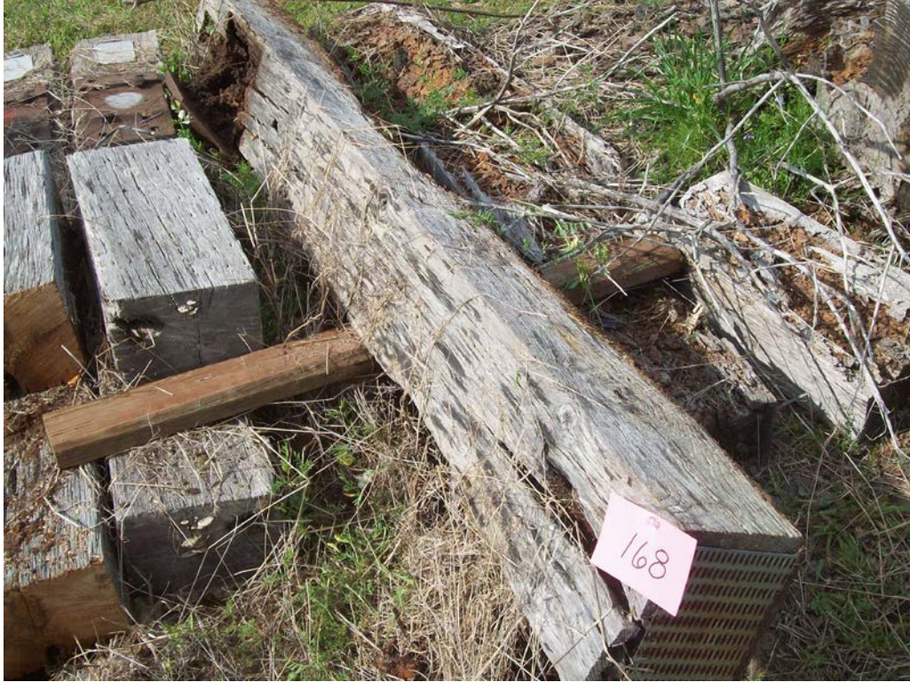
Figure 31 - Tie #168 (untreated/red oak) with decay on top and bottom.
