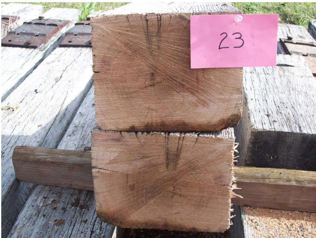
Figure 6 – Tie #23 (Envirosafe/white oak) with light decay on bottom.
