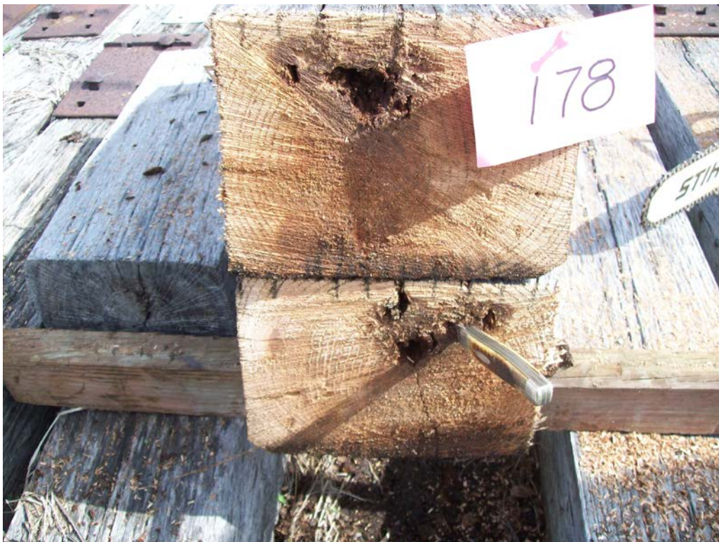
Figure 34 - Tie #178 (Lonza/red oak) with internal decay.
