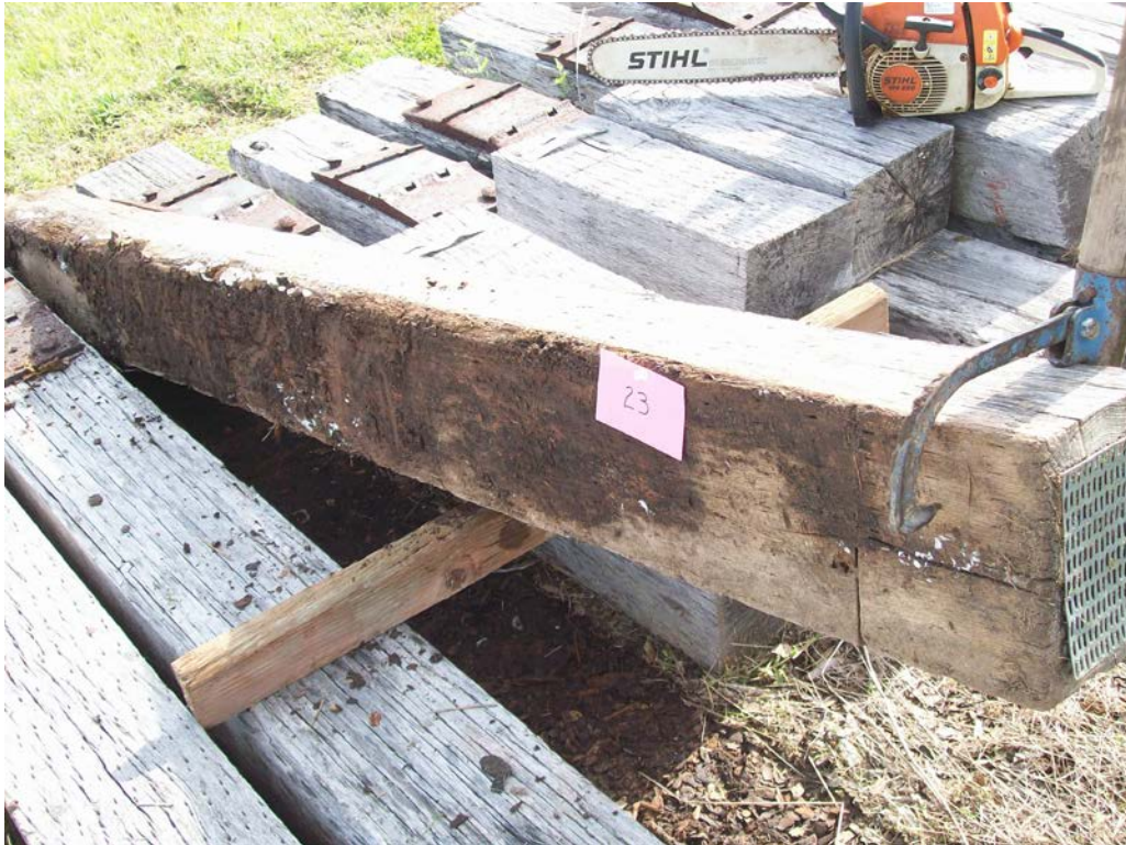
Figure 5 – Tie #23 (Envirosafe/white oak) with light decay on bottom.
