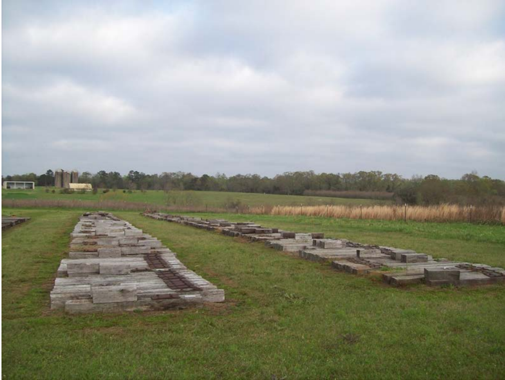
Figure 1 - An overall view of Site 2 at the time of inspection.
