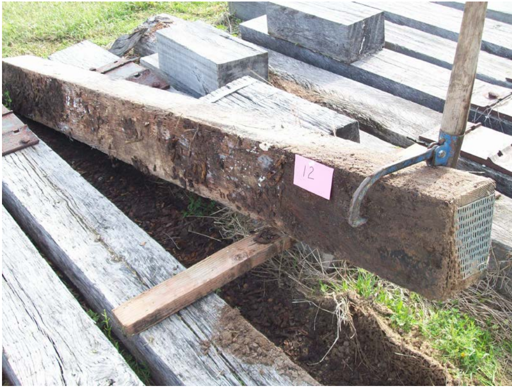
Figure 3 – Tie #12 (Envirosafe/red oak) with trace decay.
