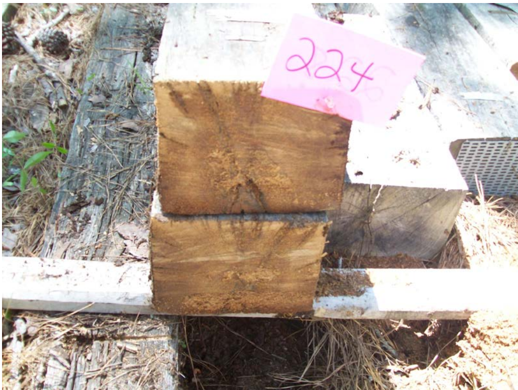
Figure 46 - Tie #224 (untreated/white oak) with decay.
