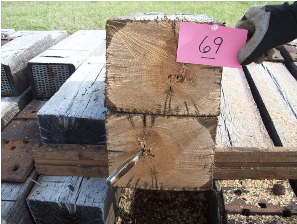
Figure 14 - Tie #69 (Boatright/white oak/borate-creosote to refusal) internal decay.
