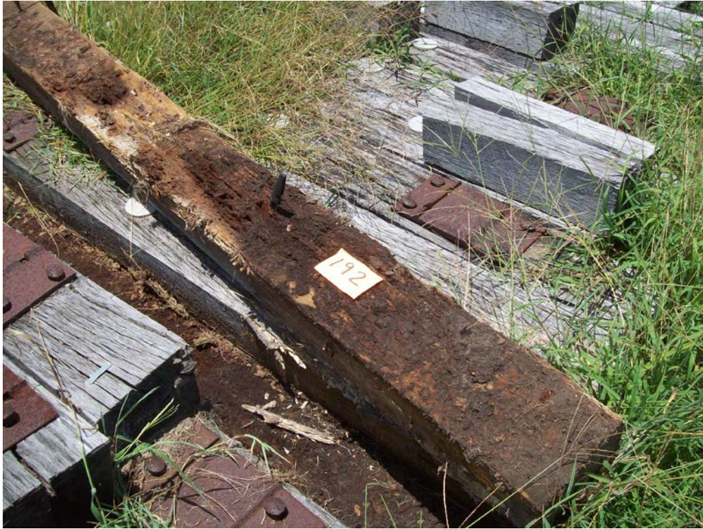
Figure 37 - Tie #192 (Cedarcide/white oak) decay on bottom and side.
