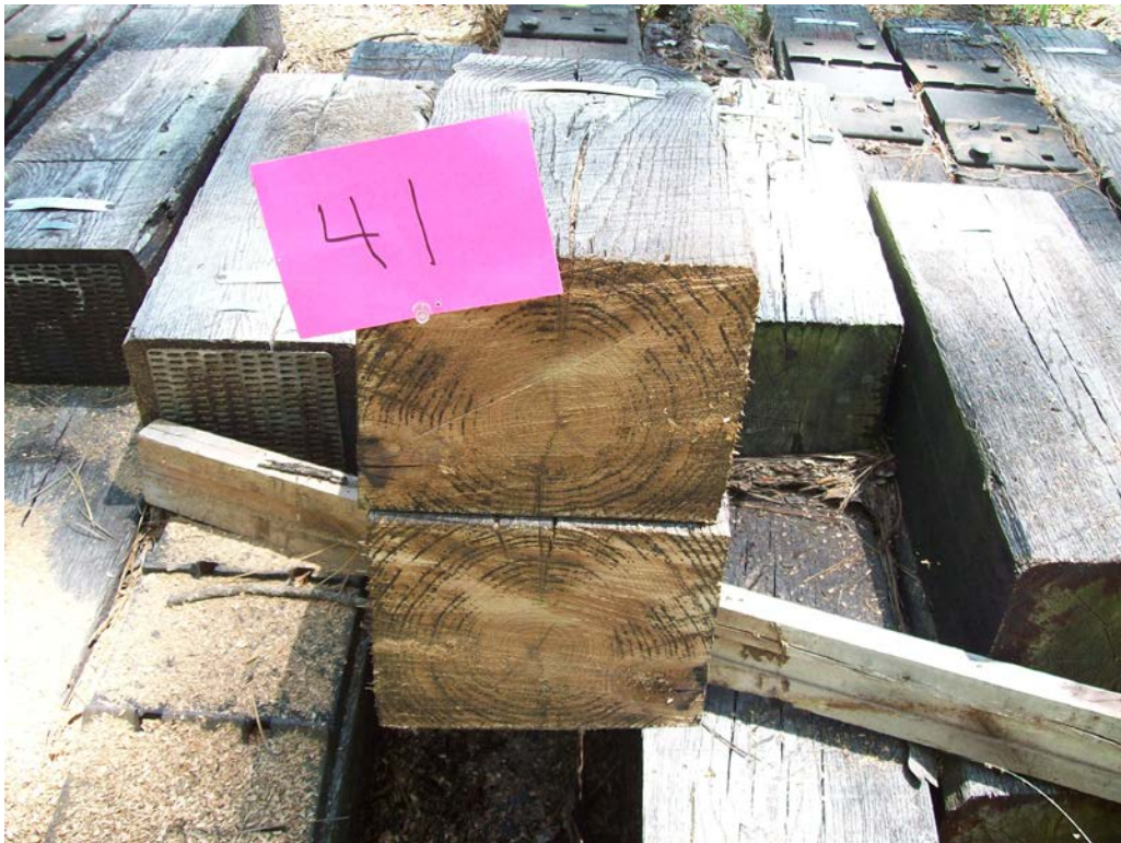
Figure 8 – Tie #33 (Boatright/red oak/borate/creosote 7pcf) internal decay around check.
