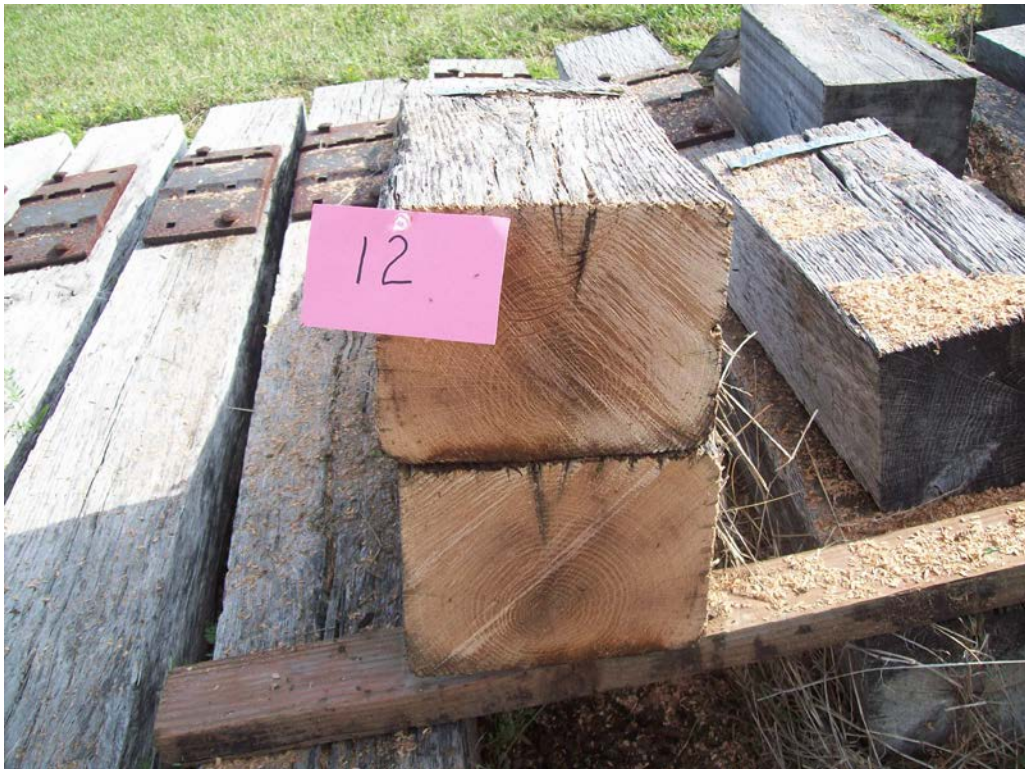
Figure 4 – Tie #12 (Envirosafe/red oak) with trace decay.
