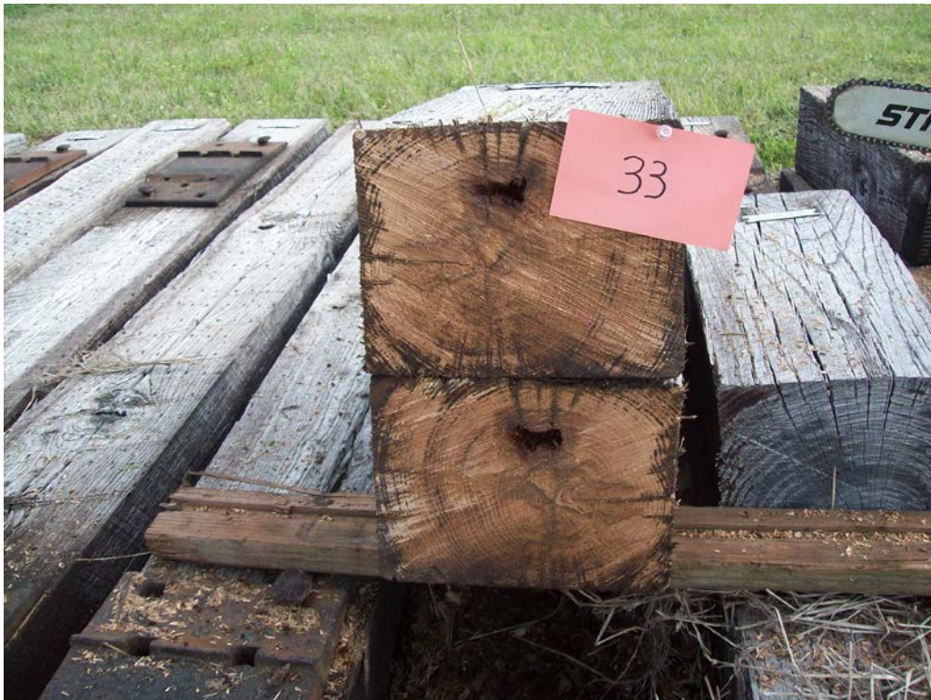
Figure 8 – Tie #33 (Boatright/red oak/creosote 5pcf) internal decay around check.
