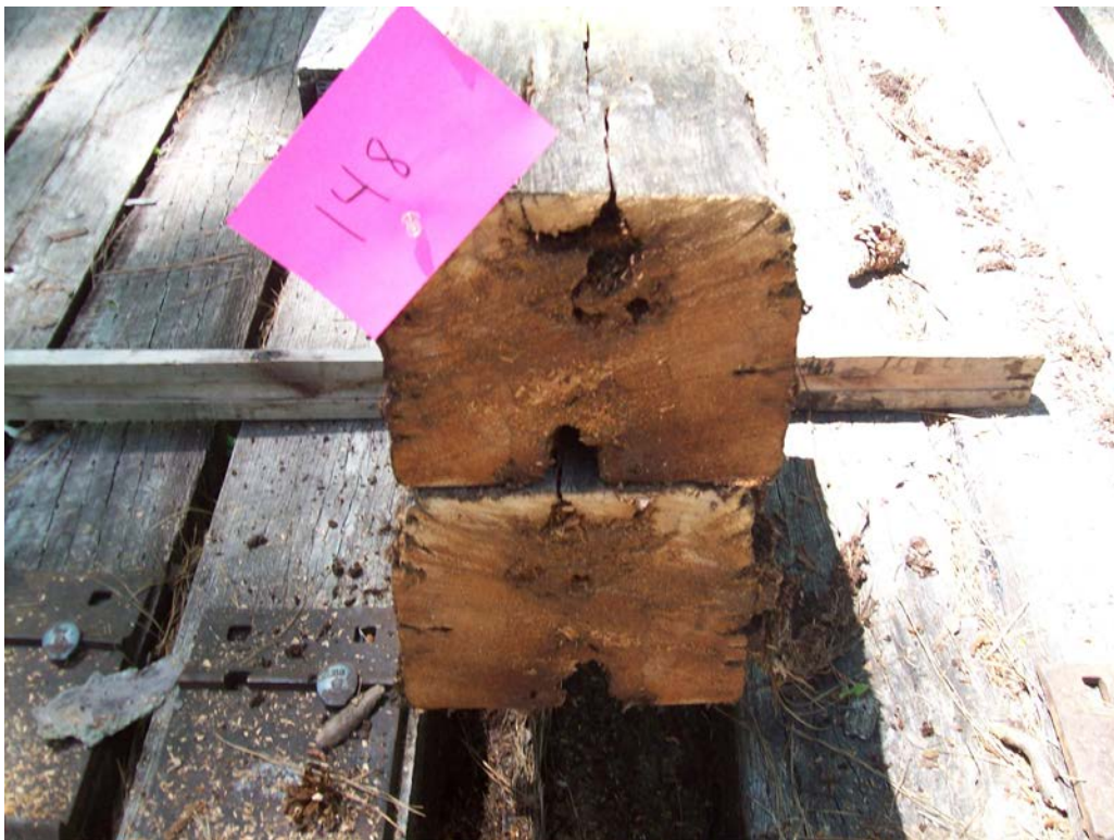
Figure 30 - Tie #148 (untreated/red oak) with extensive decay.
