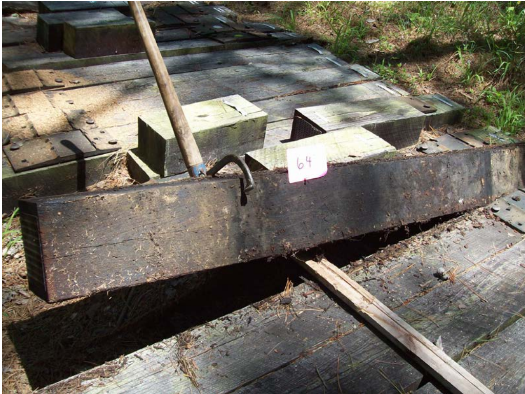
Figure 11 - Tie #64 (Boatright/red oak/creosote 5pcf).
